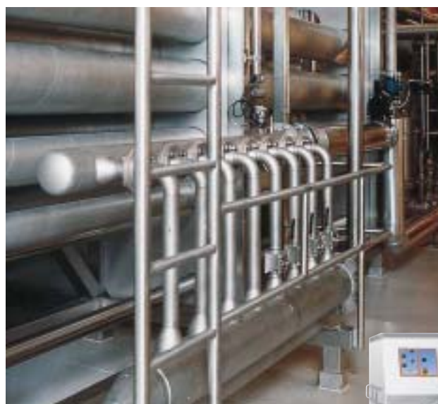
Tangential swirl heater for direct steam injection
