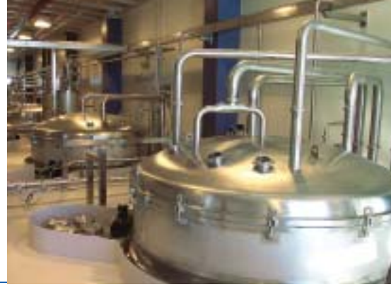
Multi-distribution system on top of calandria
