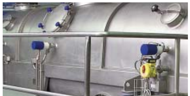
Retractable CIP-nozzle mounted on a VIBRO-FLUIDIZER®
